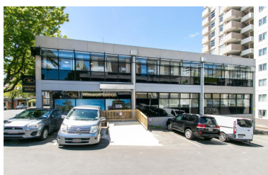
Exterior of the office
