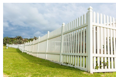
Timber Paling Fencing
